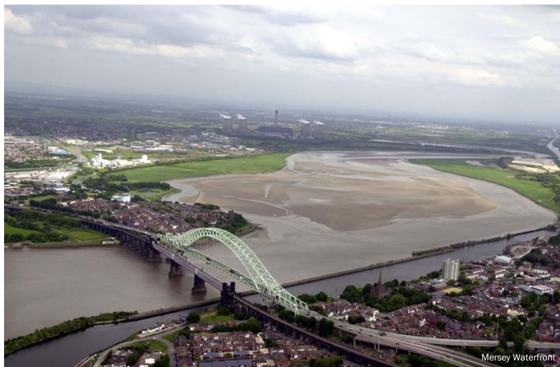
The Silver Jubilee Bridge, Halton and the Inner Mersey Estuary and Manchester Ship Canal.
