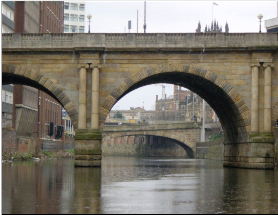
Blackfriars Bridge in 2004 - the balustrade was infilled in the 1960's, preventing views of the Irwell
